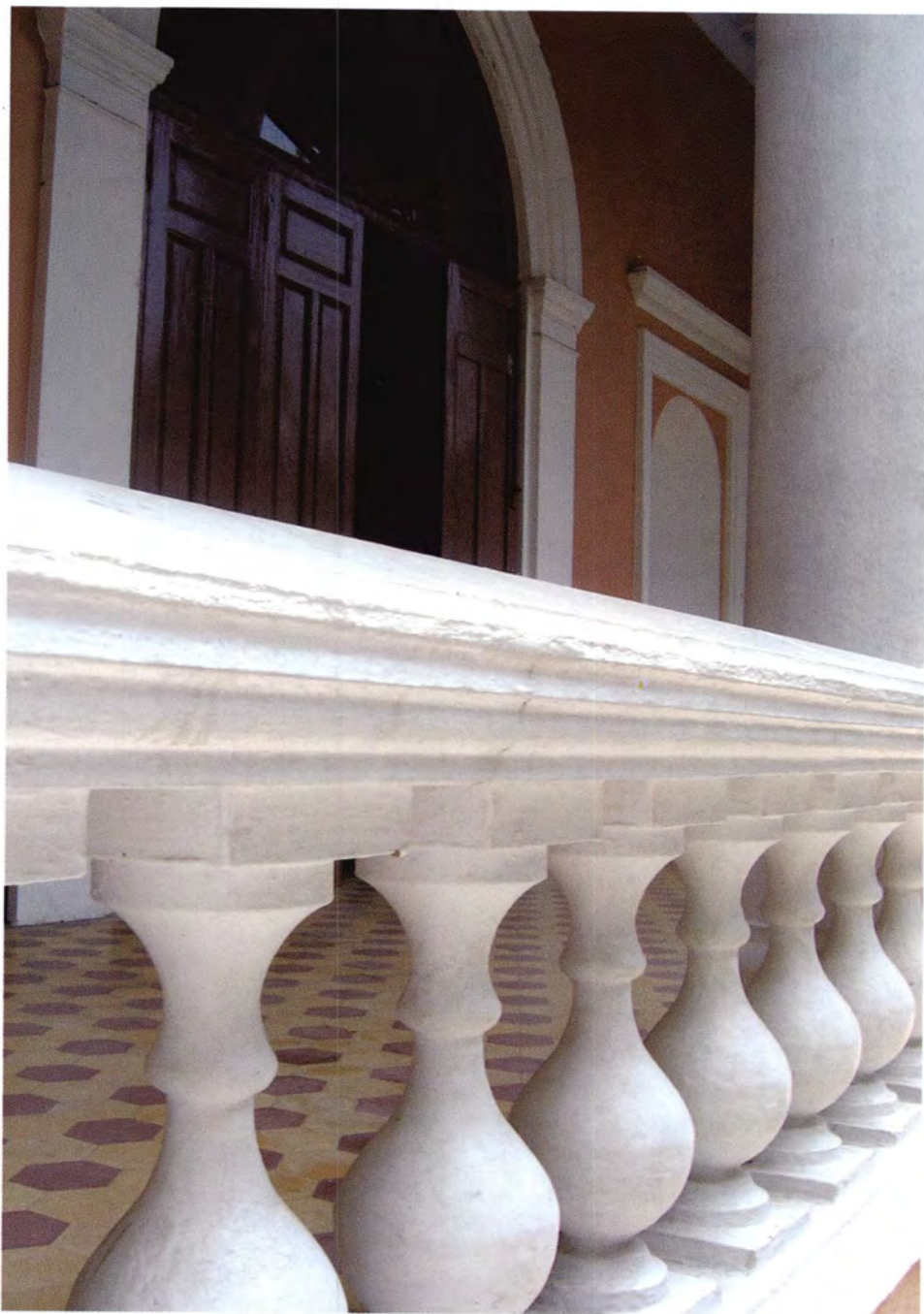
Detail of front verandah
