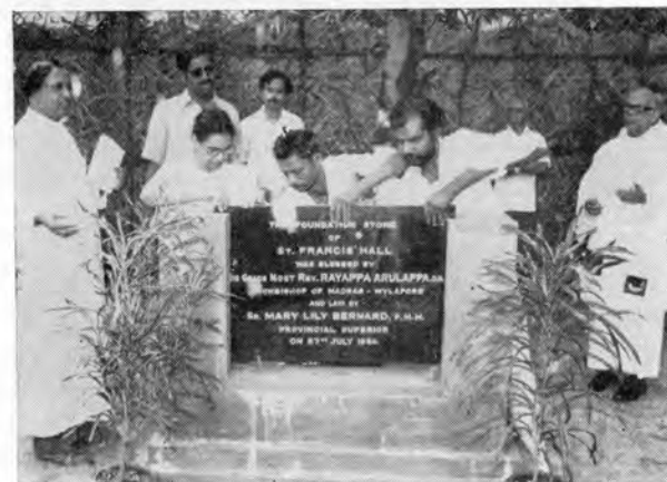
Laying the Foundation for St. Francis' Hall, our new gym.
