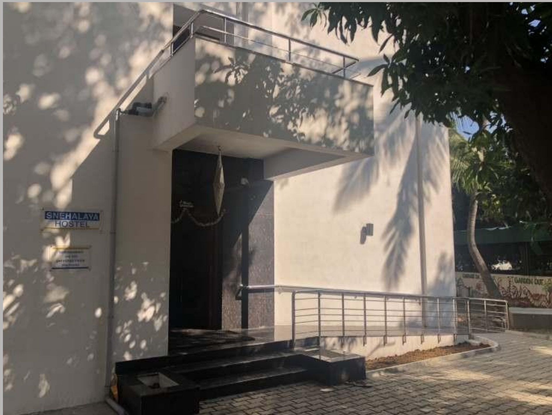
Ramp Facility at Snehalya Hostel
