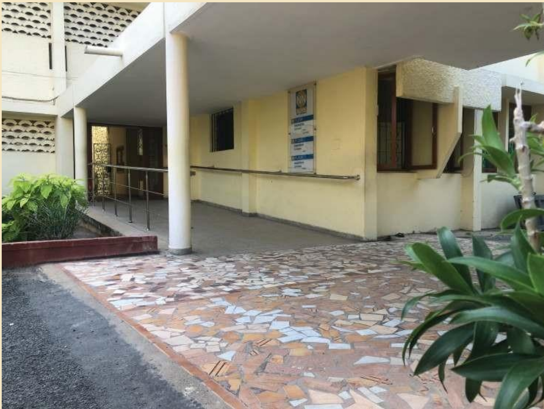
Ramp Facility at Nava Nirmana Block
