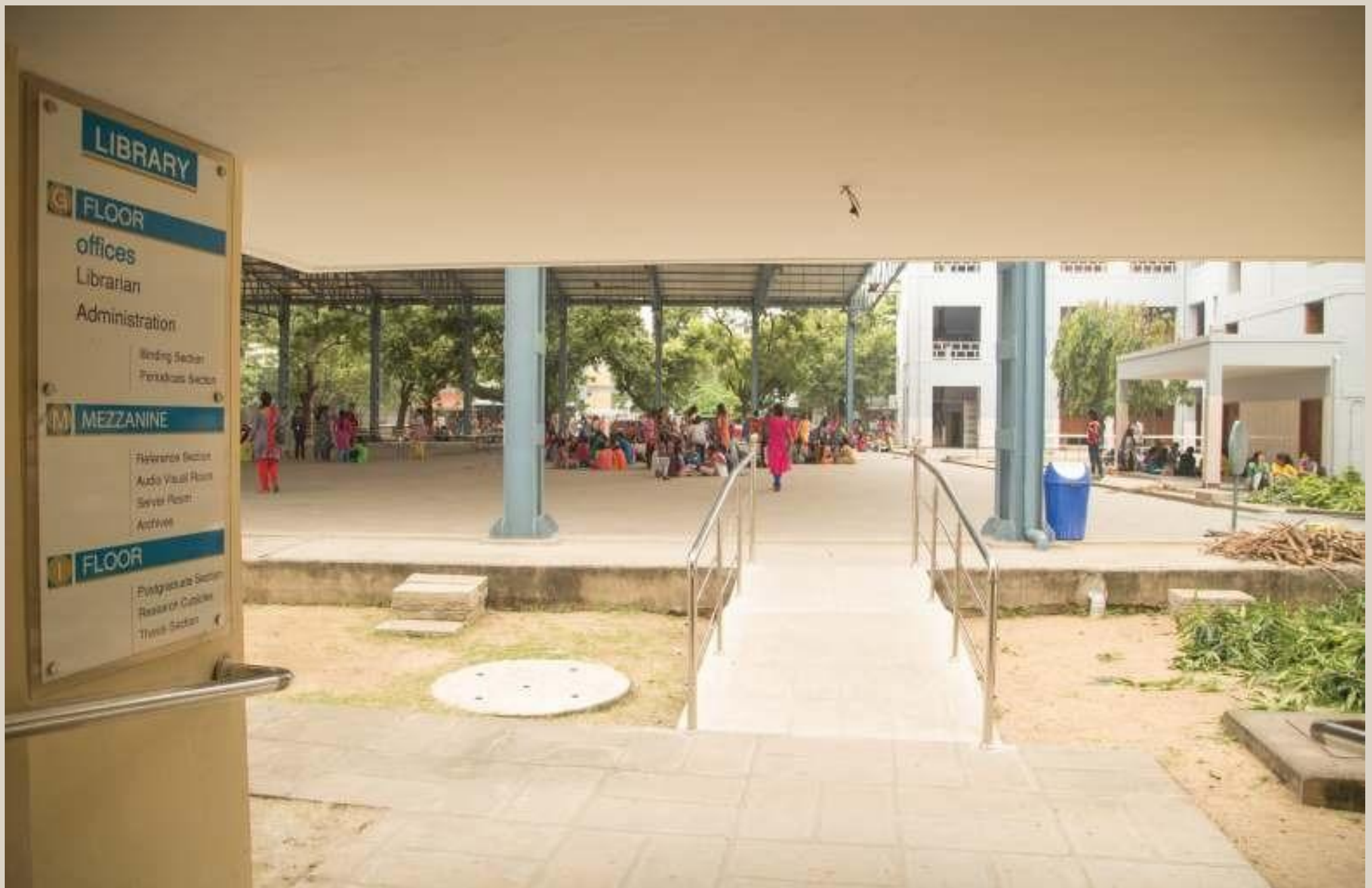
Ramp Facility to Access the College Library from the OAT
