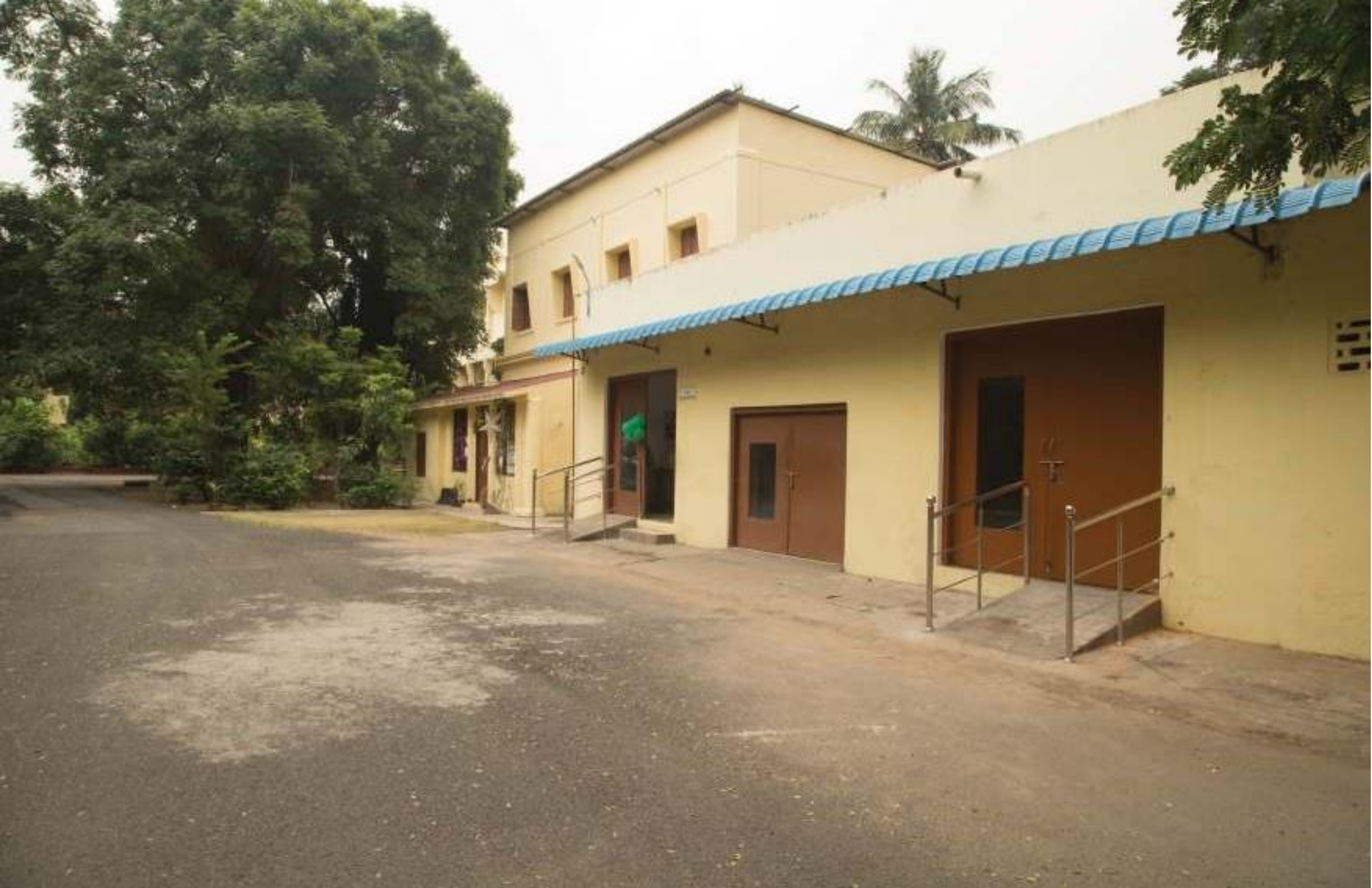
Ramp Facility at Games Room
