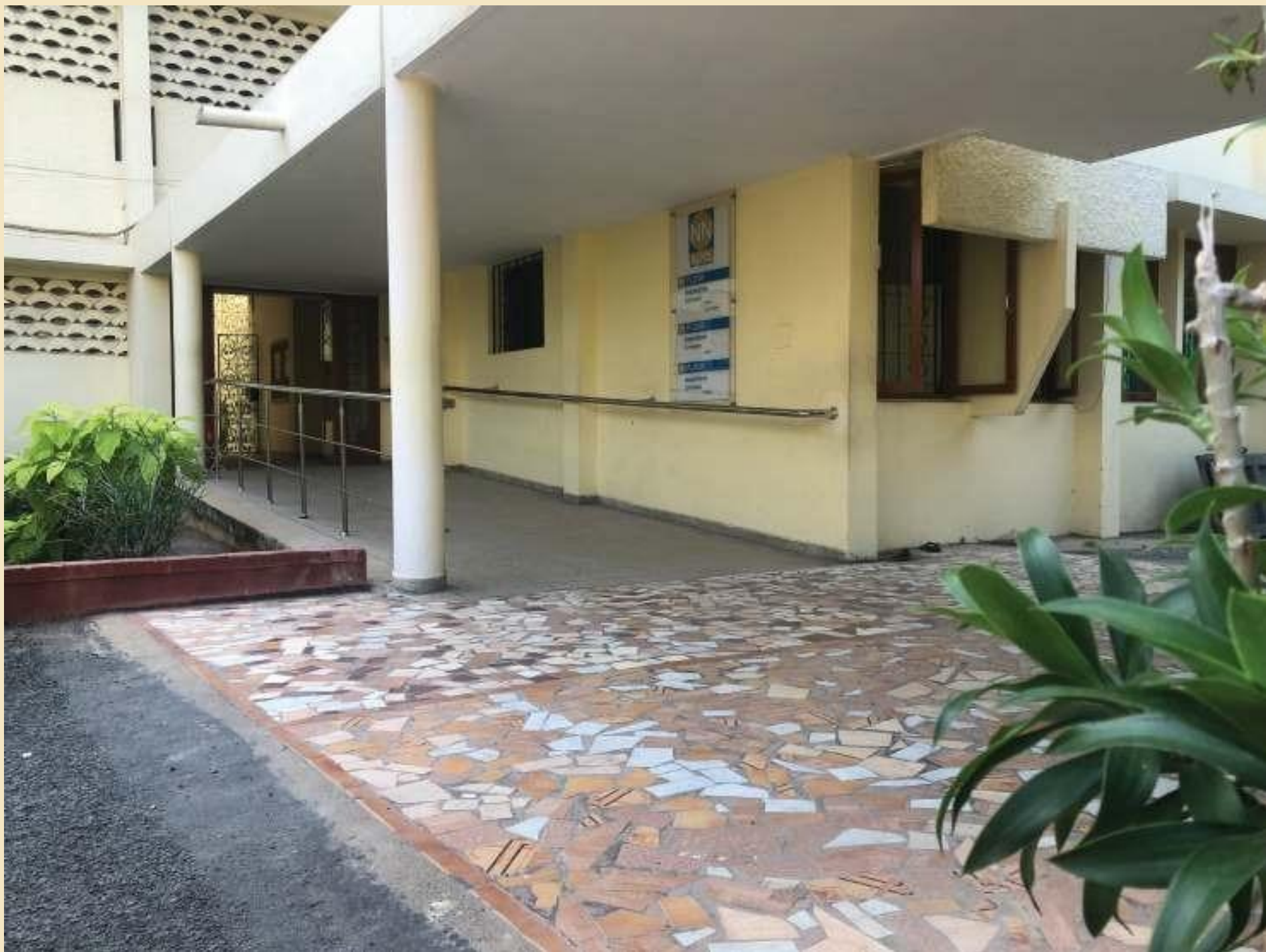
Ramp Facility at Nava Nirmana Block
