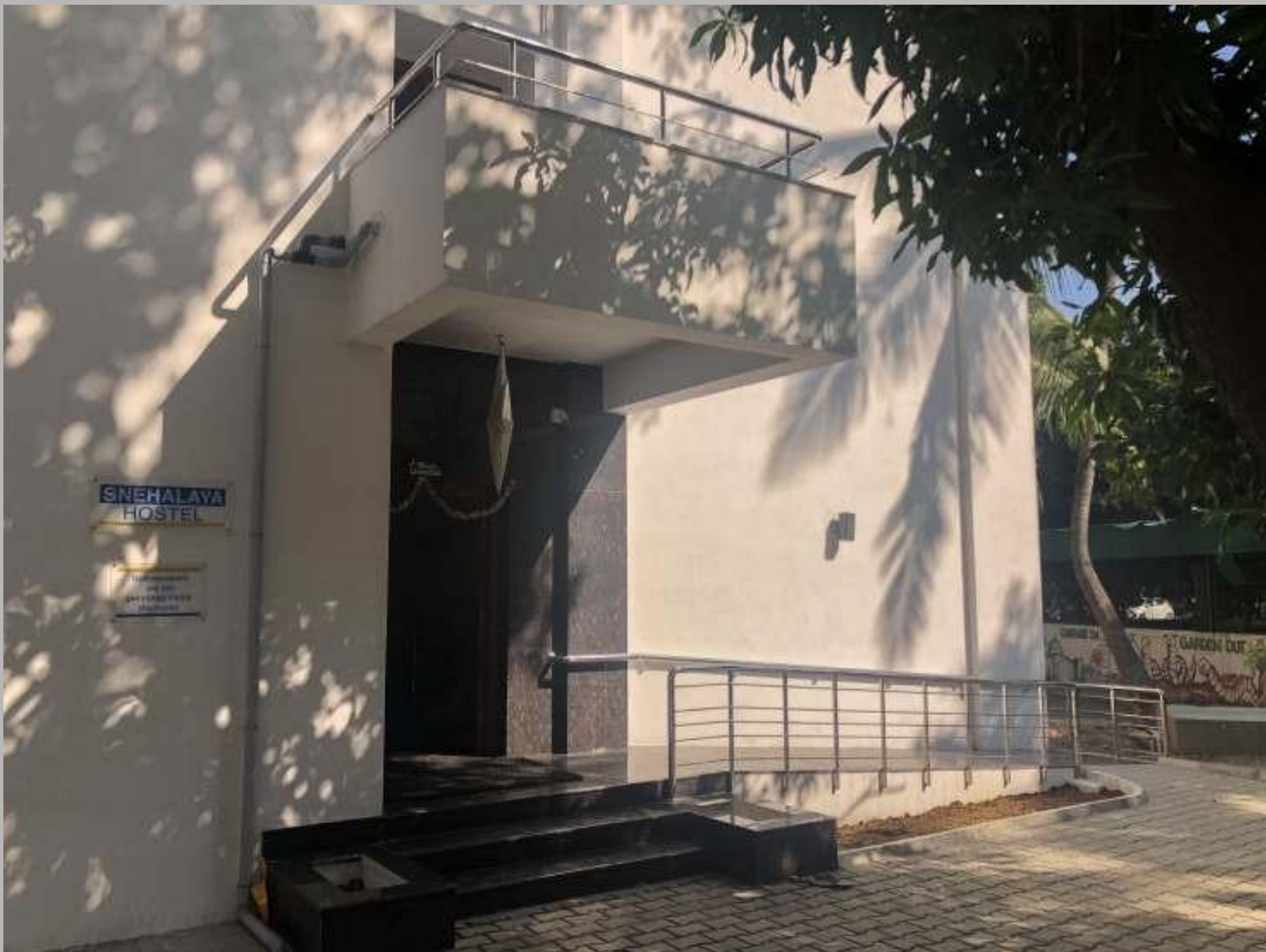
Ramp Facility at Snehalya Hostel
