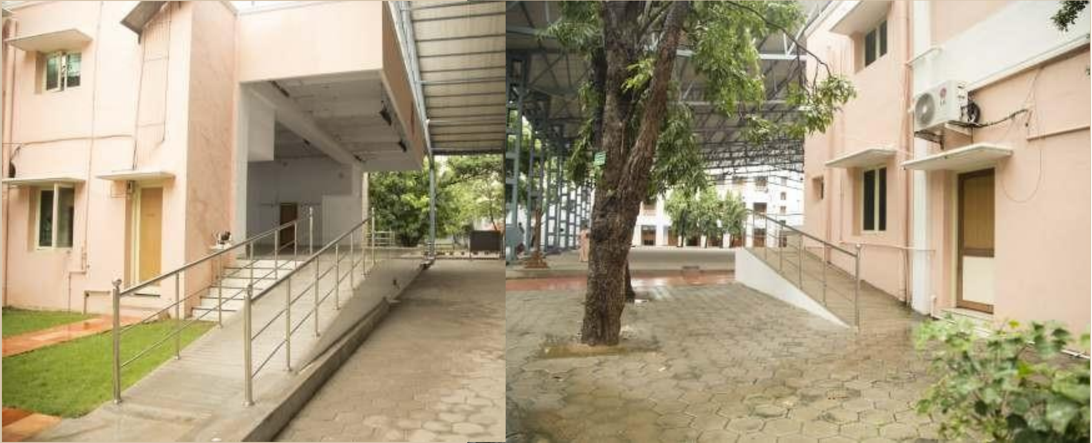
Ramp Facility for Access to OAT Stage
