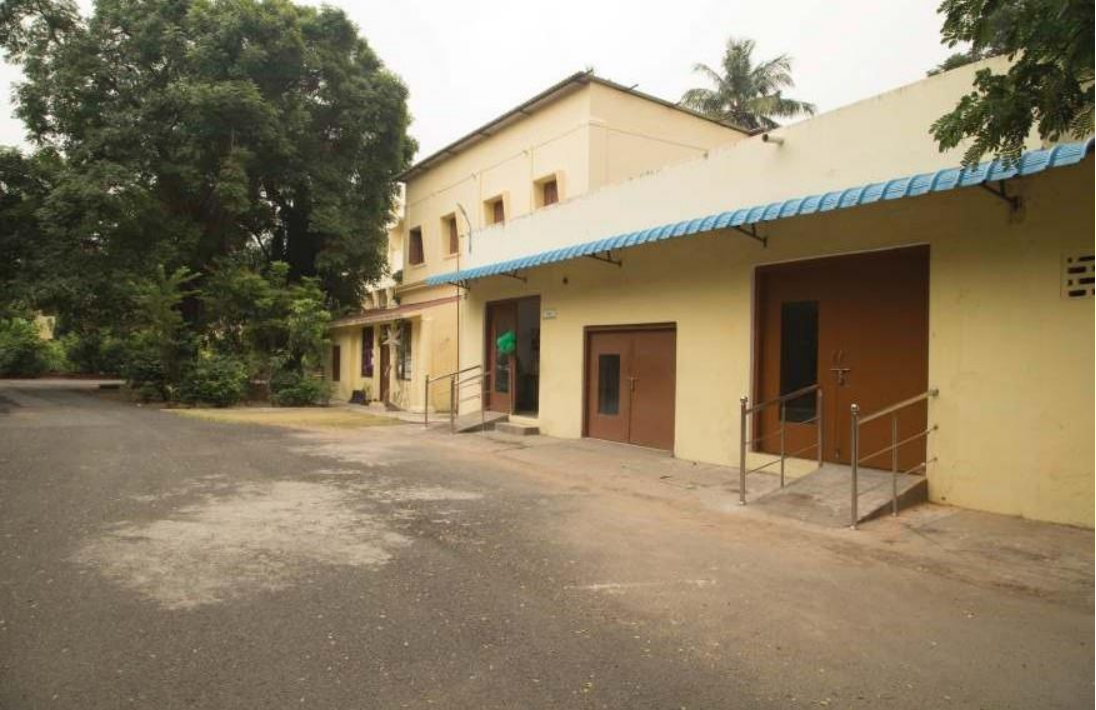
Ramp Facility at Games Room
